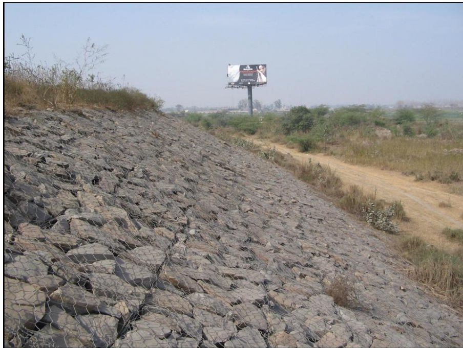
Figure 7 Existing Embankment Condition
