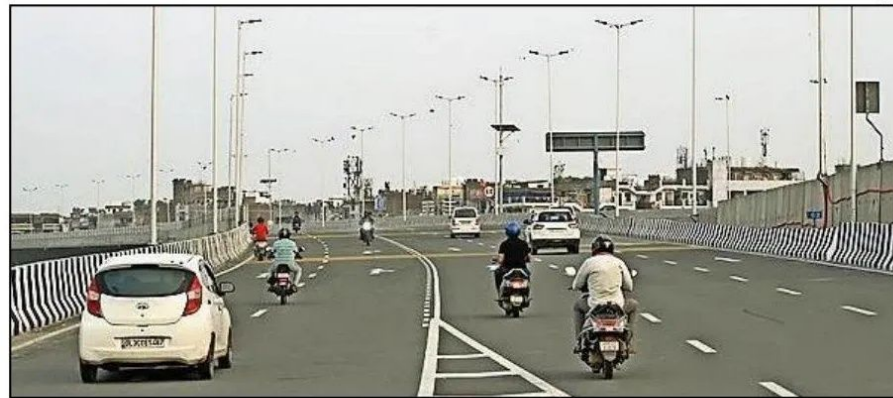
First leg of trial run on Delhi-Mumbai Expressway started on Saturday
